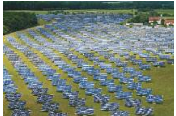
Large ground-mounted system in Germany.
