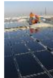
Installing thin film modules.
