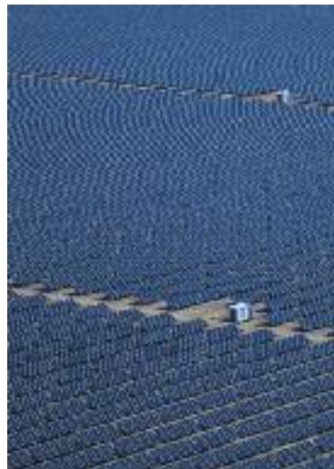
Large ground-mounted PV system in Spain.
