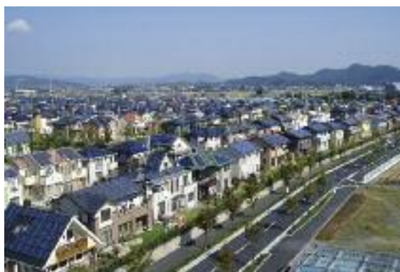
In Ohta, Japan, an interesting experiment has been conducted. The entire town has been equipped with BIPV systems to test the feasibility of a large-scale implementation.
