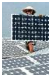
Worker installing PV on roof.
