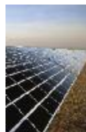
Large Thin Film power plant.
