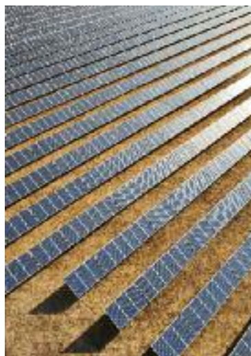
Large ground-mounted PV plant, Mallorca, Spain.
